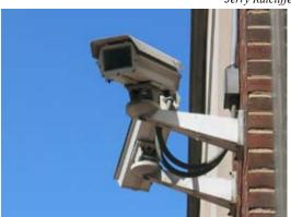
With an overt CCTV camera, the public (and offenders) can clearly see the surveillance camera and determine the direction in which it is facing.
